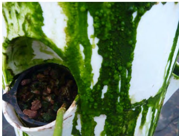
Fig 3.9 Algae Growing on PVC Pipe
