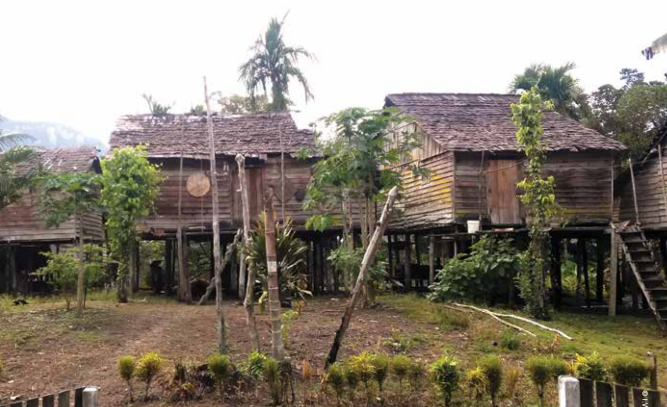
Housing raised on stilts for protection from floods and wild animals (Indonesia).
