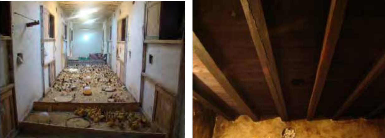
Photo 4 Recently built TH (hatched DOBs in Qasaba –left)
