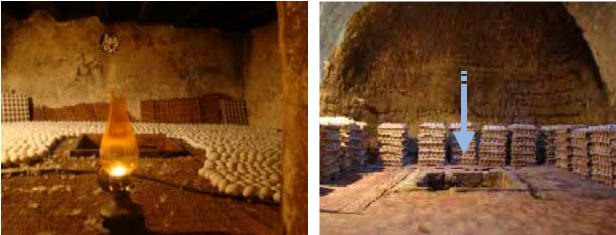
Photo 2 Upper unit of egg house, notice central manhole to the lower unit, feathers and egg racks.
