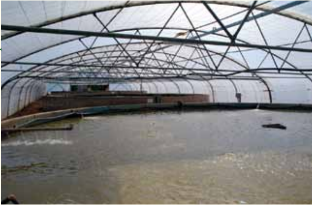
Concrete tanks inside a greenhouse in the Hardap Inland Aquaculture Centre
