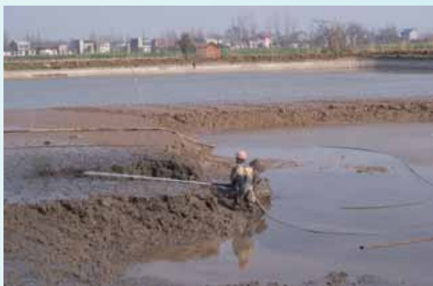
Desiltation of ponds in progress
