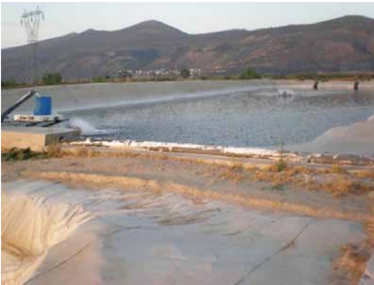
Figure 28: Earthen ponds with their beds covered by a geomembrane.
