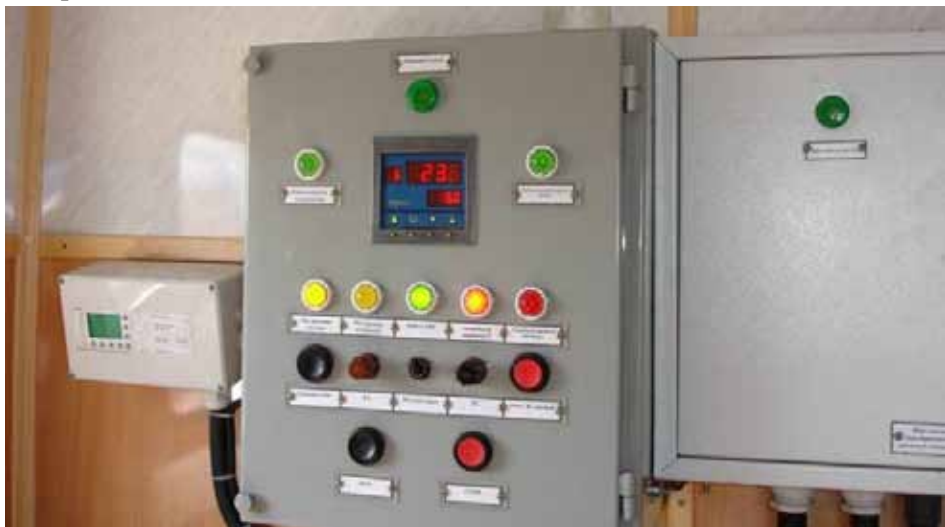
Figure 112: System to control temperature and oxygen of transport water (Chepurkina et al. , 2008).
