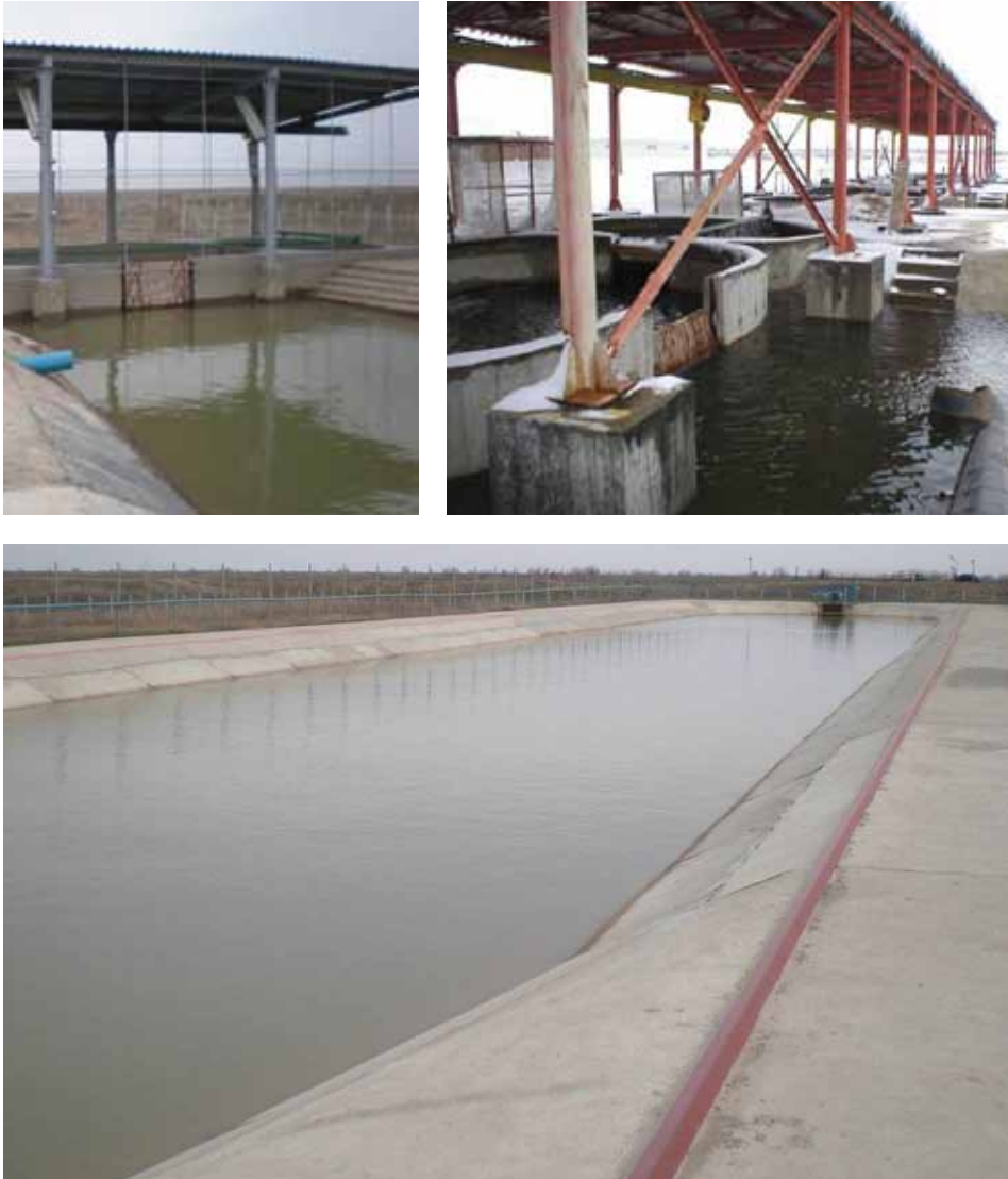
Figure 24: Pond facility of the “Kurinsky” type.
