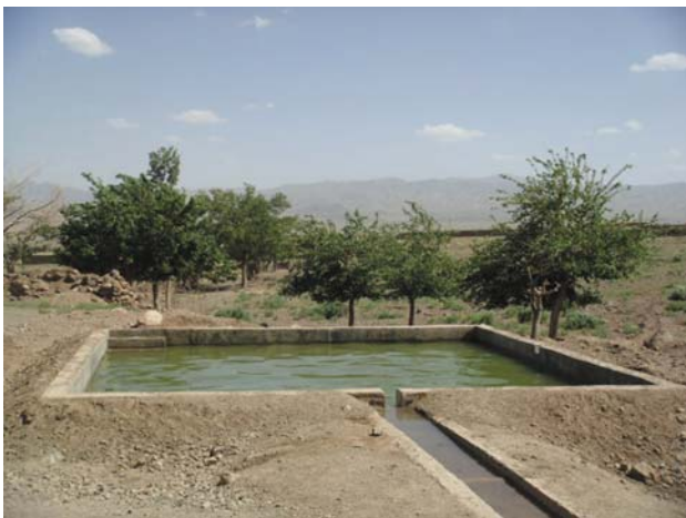
Figure 2. Sheikh Umar Karez village water storage after improvement undertaken by the Community Organization who contributed 50 percent of the costs. Water flow also increased due to cleaning and extension of the Karez system.
