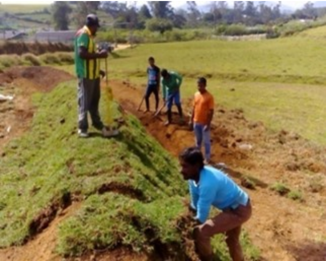
Multi purpose earth bunds
