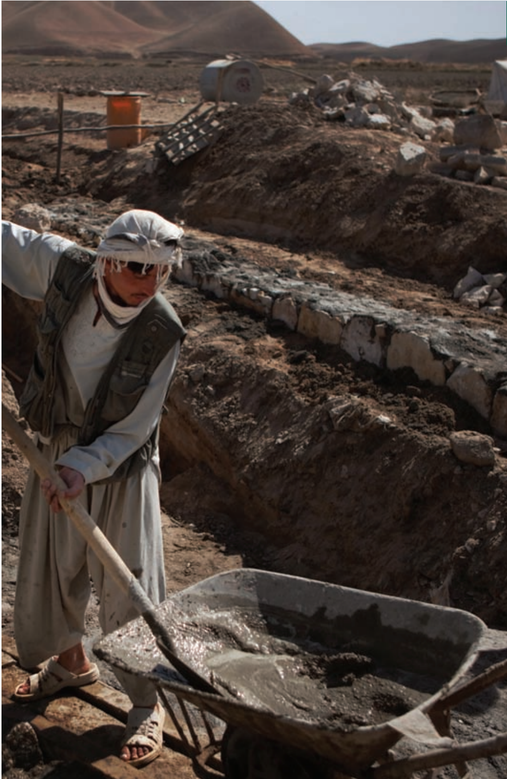
Workmen constructing an irrigation channel, Afghanistan.
