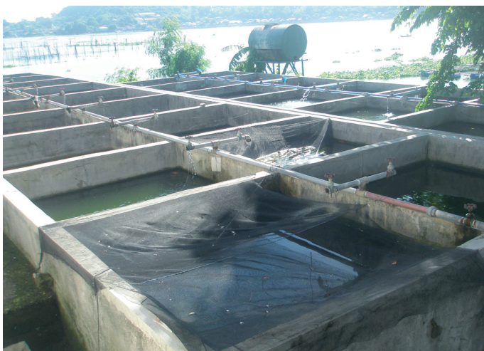
FIGURE 1.4 Concrete tanks for use in breeding and small-scale tilapia farming
