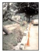
installed. If pavement displacement is less than one inch, grinding down the edge of the raised surface can be an effective solution.
