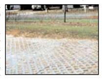
leable paving surfaces that give way to invasive tree roots. Rubber sidewalks are cost-effective and aesthetically acceptable alternatives to conventional paving materials. Though rubber sidewalks may bend a bit out of shape in response to aggressive roots they do not create abrupt edges over which pedestrians might trip, and they provide a softer surface should someone fall on them.
