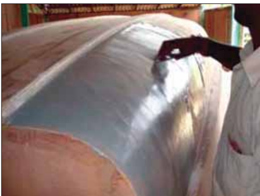
Figure 51 Applying autograde putty.
