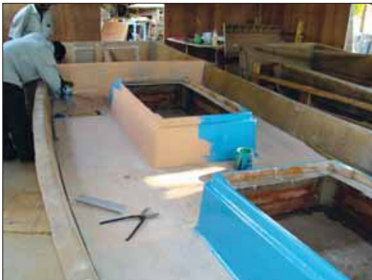
Figure 106 Topcoat being applied.
