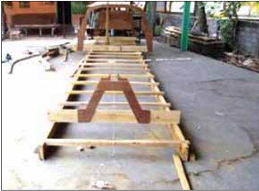
Figure 43 Frame assembly on jig.
