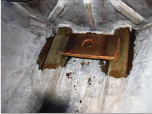
Figure 116 The mast step.
