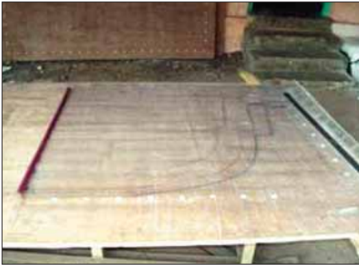
Figure 41 Lofting on plywood – mylar film transfer.
