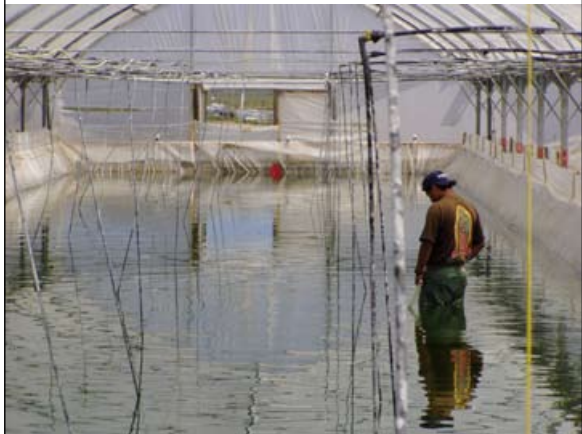
PHOTO 34 Rectangular tanks covered with PVC in Baja California
