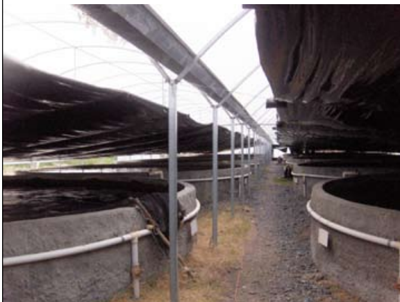
PHOTO 35 Concrete tanks covered with PVC against solar radiations
