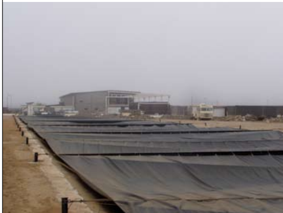
PHOTO 33 Hatchery and tanks covered with liners to avoid sand contamination in Baja California
