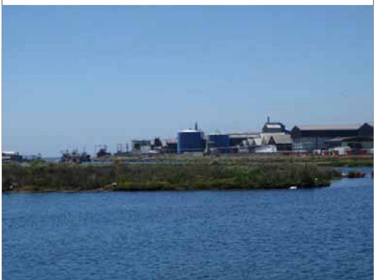
Fishmeal and fish oil processing factory in Talcahuano, Chile
