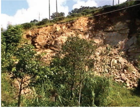
Landslide on Monteviot tea estate (close view)
