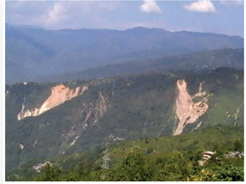
Landslides on tea estates (distant view)
