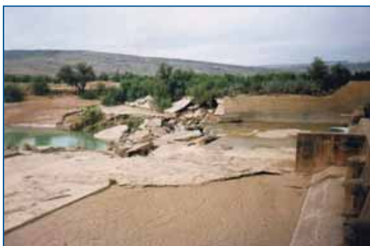
FIGURE 7.5 Diversion weir blown up by farmers as it interfered with the base flows, Pakistan
