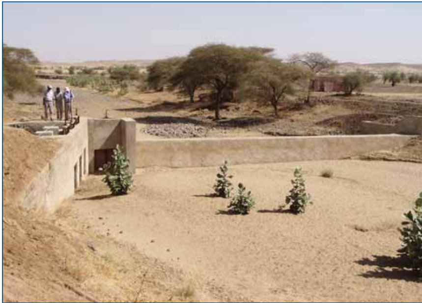
FIGURE 4.19 Adurguyay intake, Eritrea
