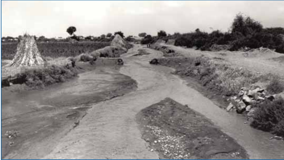
FIGURE 4.20 Traditional canal diversion bund, Wadi Zabid, Yemen
