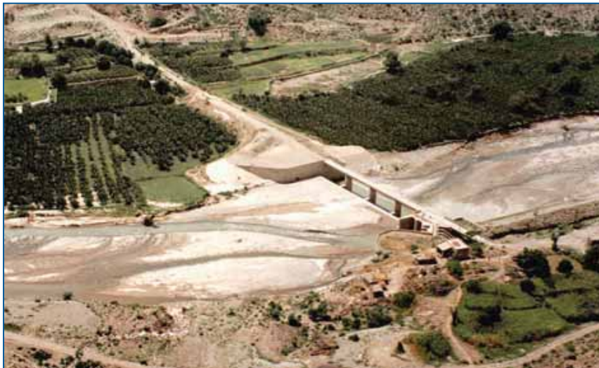
FIGURE 4.15 Wadi Rima spate irrigation intake, Yemen
