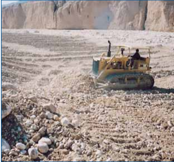
FIGURE 4.11 Diversion bunds under construction using a bulldozer in Pakistan
