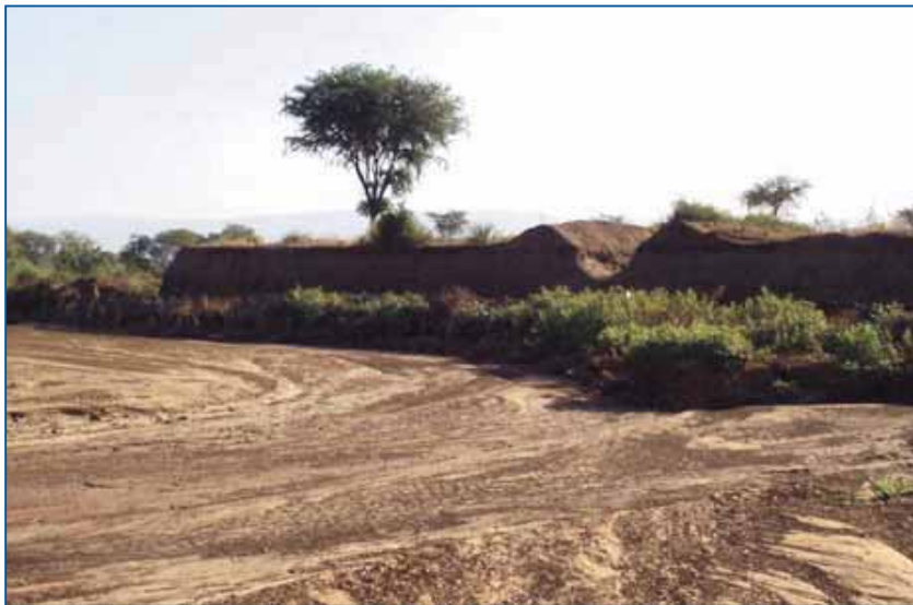
FIGURE 10.2 Lowered river bed and eroded river banks causing the abandonment of the canal head, Ethiopia
