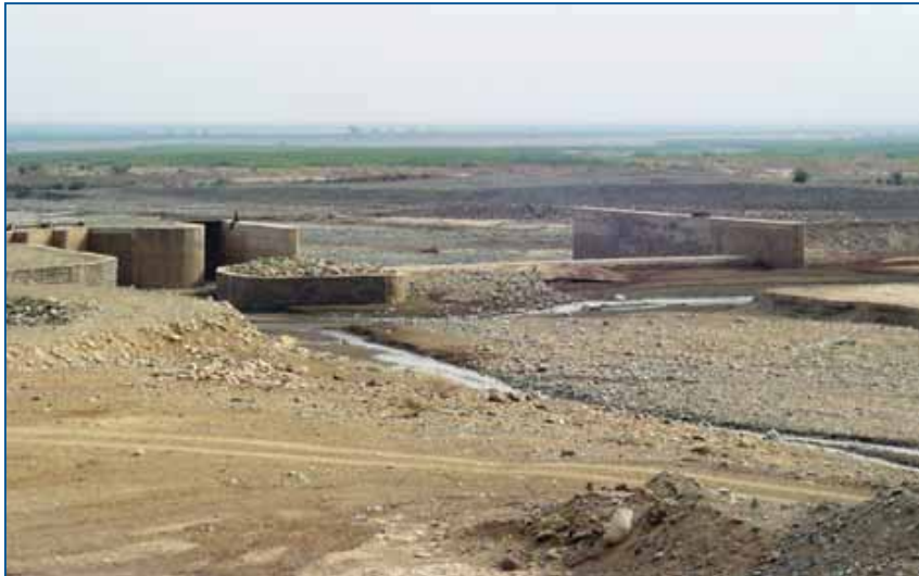
FIGURE 4.18 Spate diversion structure constructed at Wadi Laba in Eritrea
