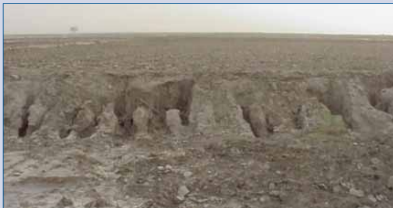
Severly eroded field bund in Wadi Laba, Eritrea ( Mehari et al., 2005b )
