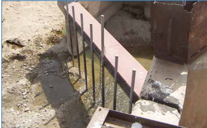
FIGURE 4.17 Trash deflector, Wadi Rima intake (2003)
