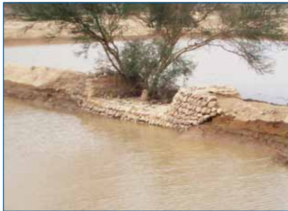
FIGURE 5.6 Stone reinforced field-to-field intake structure in Pakistan
