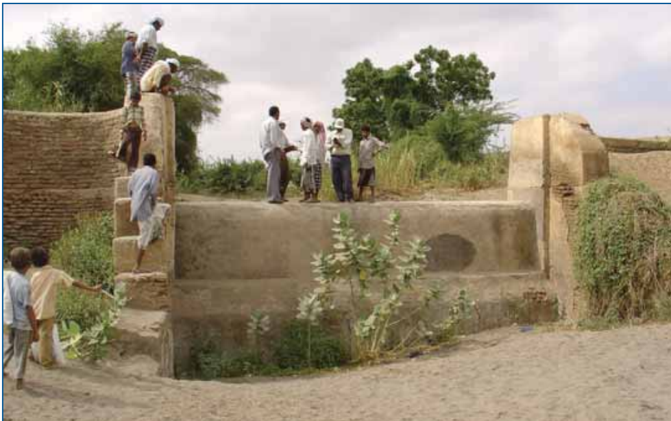
FIGURE 4.21 Stepped drop structure, Wadi Zabid, Yemen
