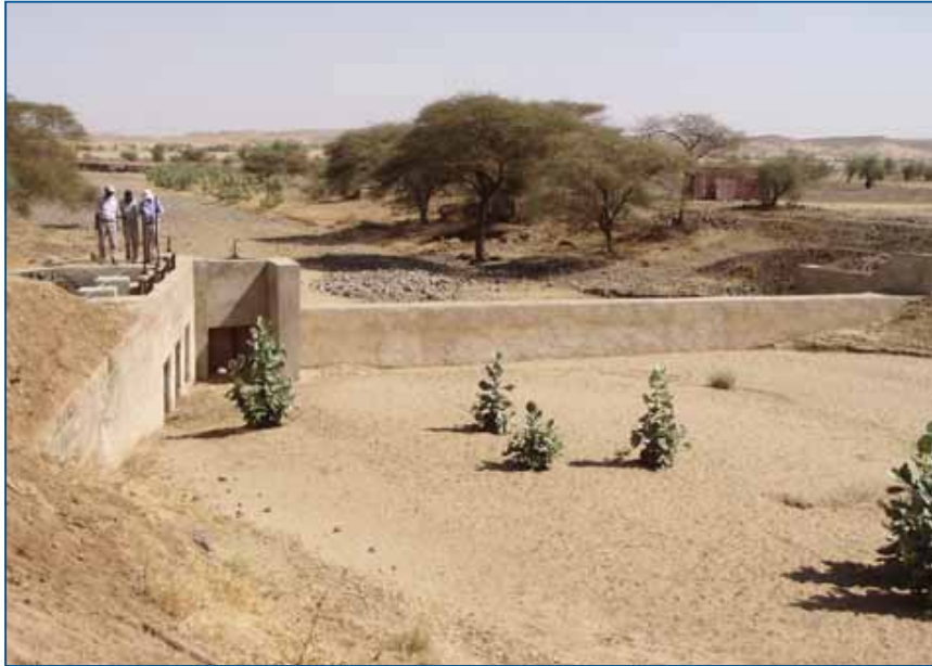
FIGURE 4.19 Adurguyay intake, Eritrea
