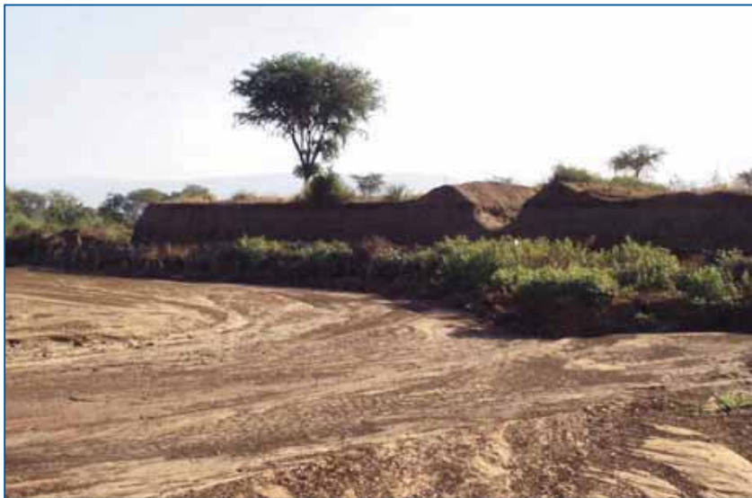
FIGURE 10.2 Lowered river bed and eroded river banks causing the abandonment of the canal head, Ethiopia
