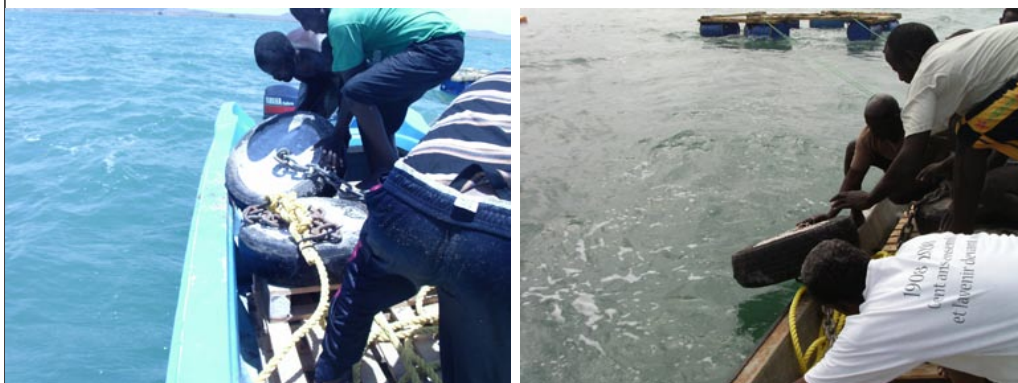
PLATE 38 Lowering the mooring posts into the sea
