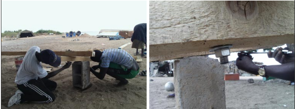
PLATE 24 Tightening of screws
