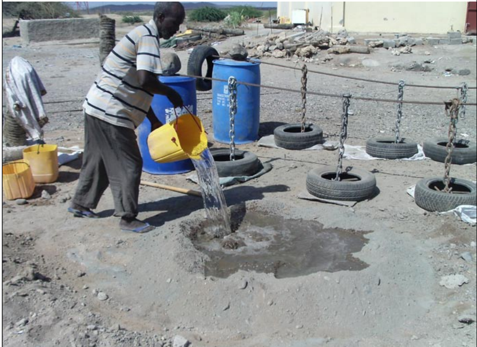
PLATE A3.1 Mixing concrete
