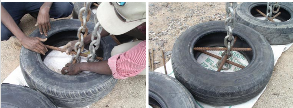
PLATE 15 Crossed iron bars in the tyres
