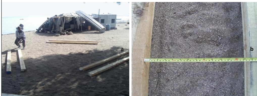
PLATE 19 (a) Arrangement of the first lower beams; (b) verification of the distance between the parallel beams
