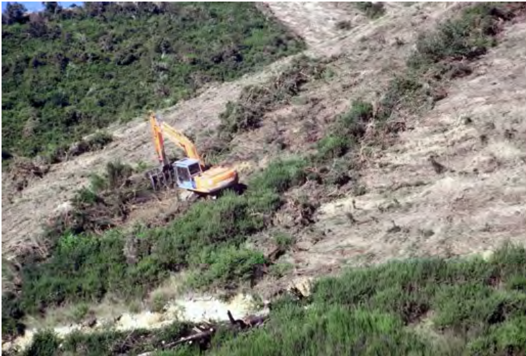
FIGURE 8.5 Windrows made using a backhoe with a root-rake attachment. Note that there is some soil disturbance.
