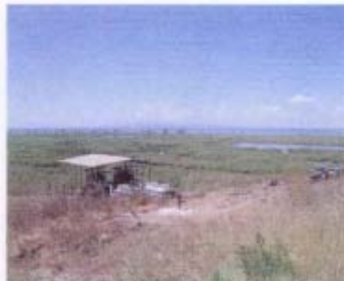
Photo 15. Kapishi Geothermal Plant, Zambia
