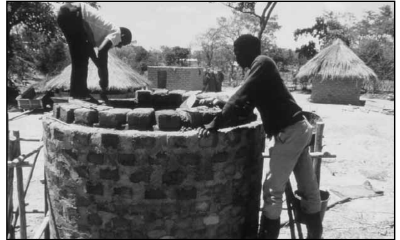
Beginning to inset top bricks to form roof
