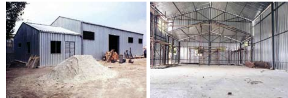
FIGURE 39 All-metal workshop under construction
