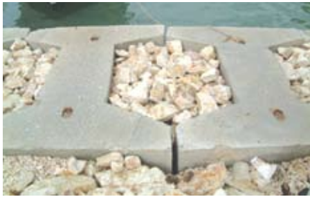
FIGURE 28 "I" blocks in-filled with rock
