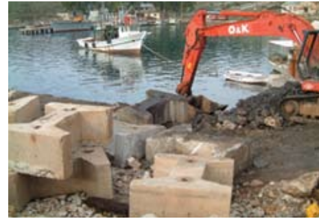
FIGURE 27 "I" section blocks (10 tonnes)
