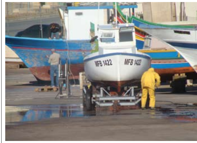
FIGURE 42 Power washing hull
