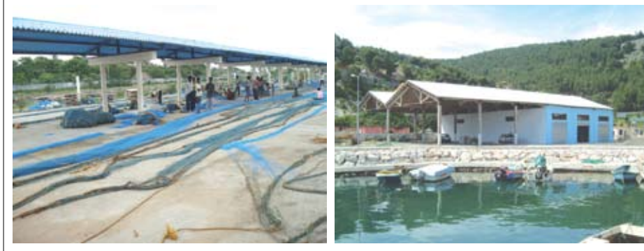
FIGURE 43 Large-scale net repair structures
