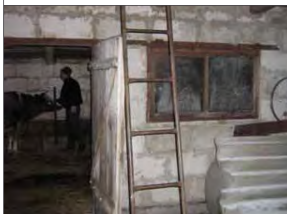
Picture 3. Foam concrete block barn
