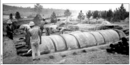
A semi-permanent low-cost "Subrifosse" type metal kiln in Madagascar was designed to carbonize offcuts from sawmilling
