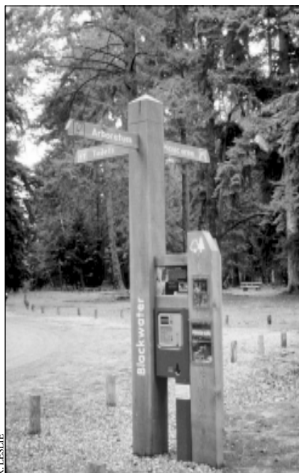
A car-park meter combined with an information point, chunkily built from wood to look good in the forest and resist damage
