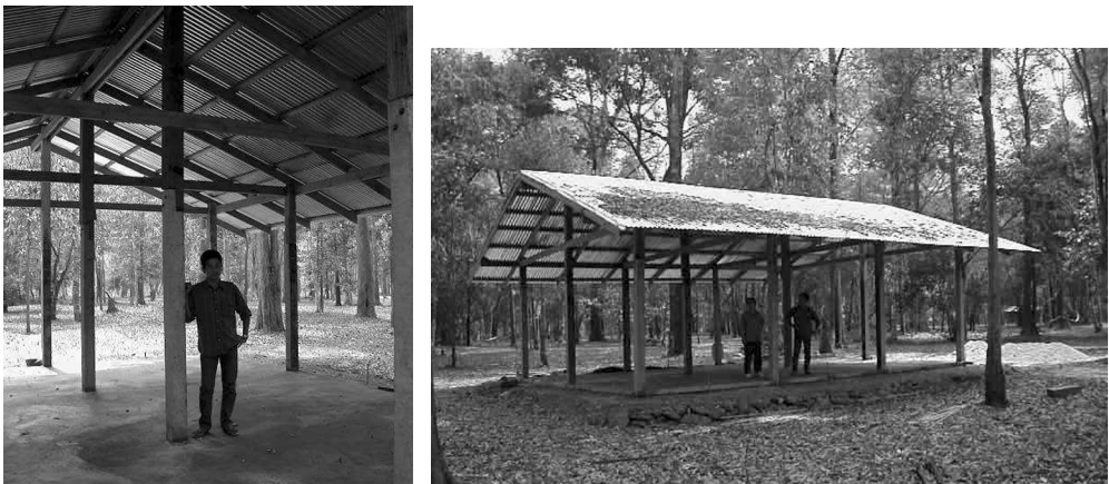
Figure 7. The public hall under construction
