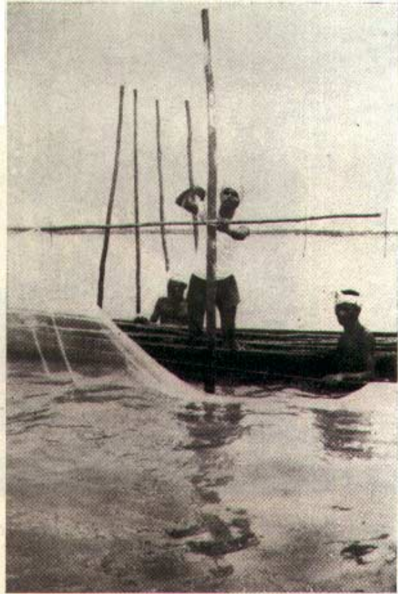
Right: Erection of pens.
