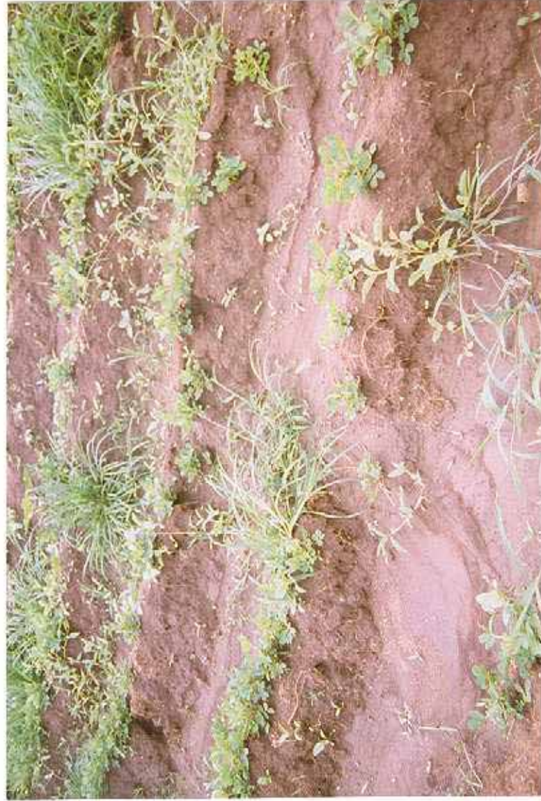
Photograph 3. Crop ridge breakage as rainfall unable to infiltrate due to the presence of a hoe pan, Nathenje, March 1999
