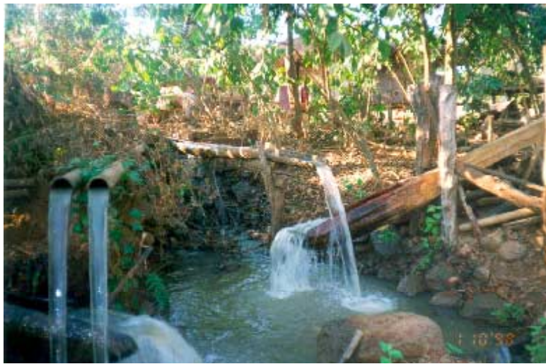
Figure 2. Excellent water source from clear-water stream (dry season flow)
