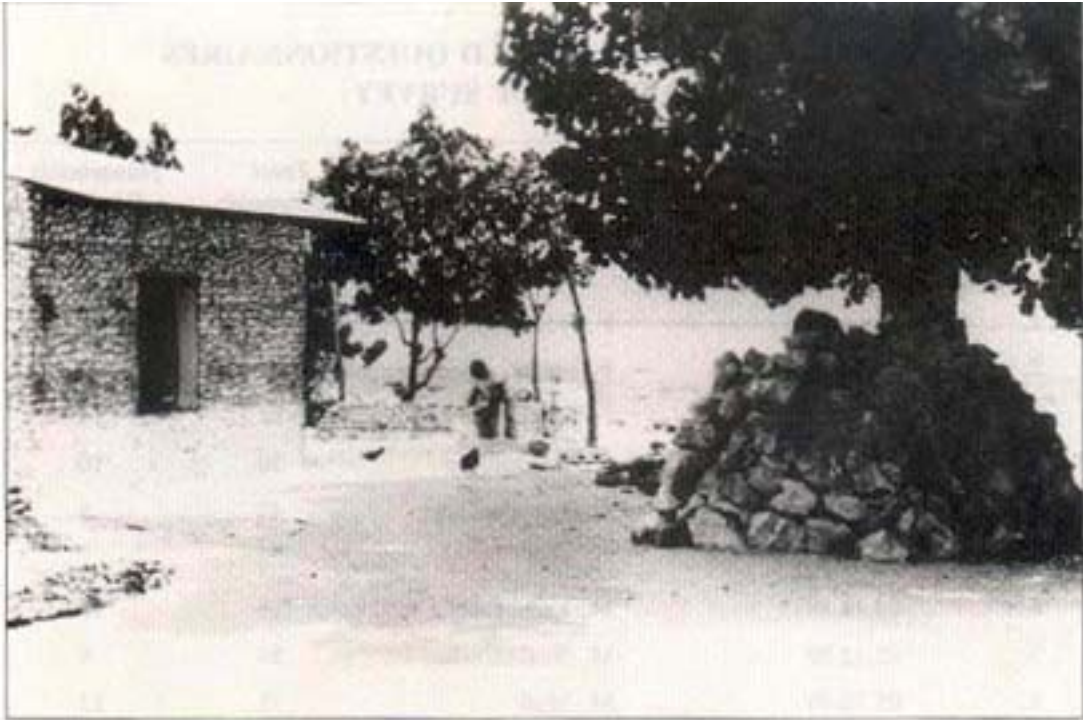
Building a house with bits of the coral reef in the Maldives
