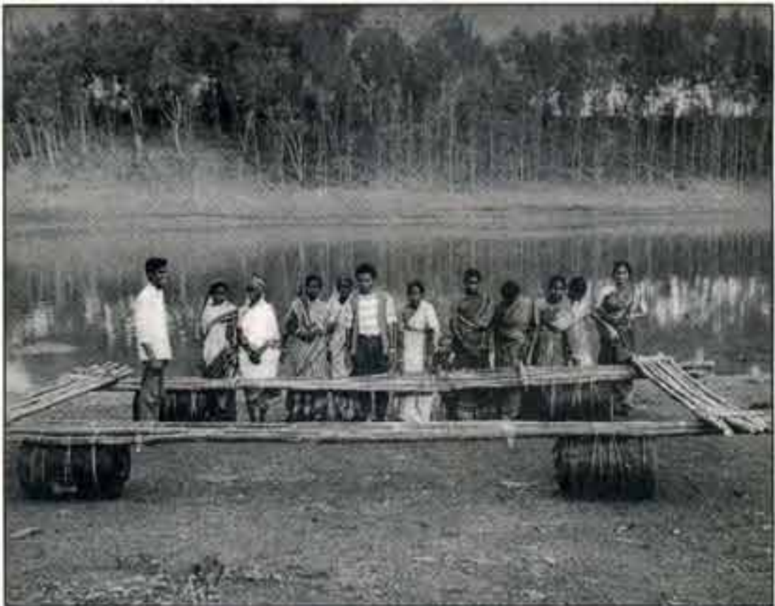
The complete cage frame ready for launching
