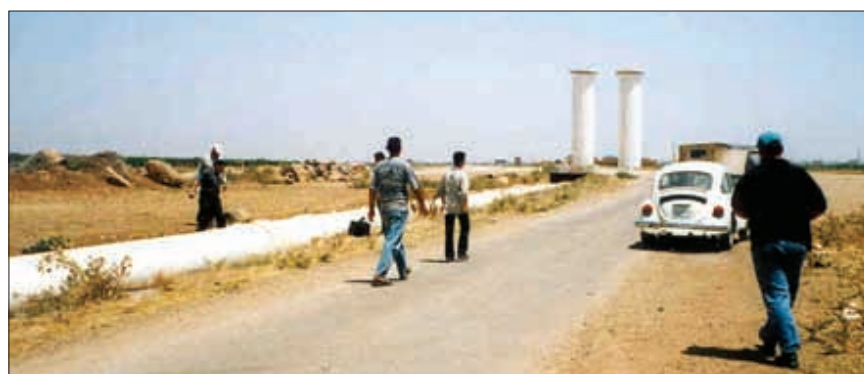
Old Alyarmook Project, Alyarmook Basin, Southern Syria Conveyance system after modernization (pressurized pipe system).
