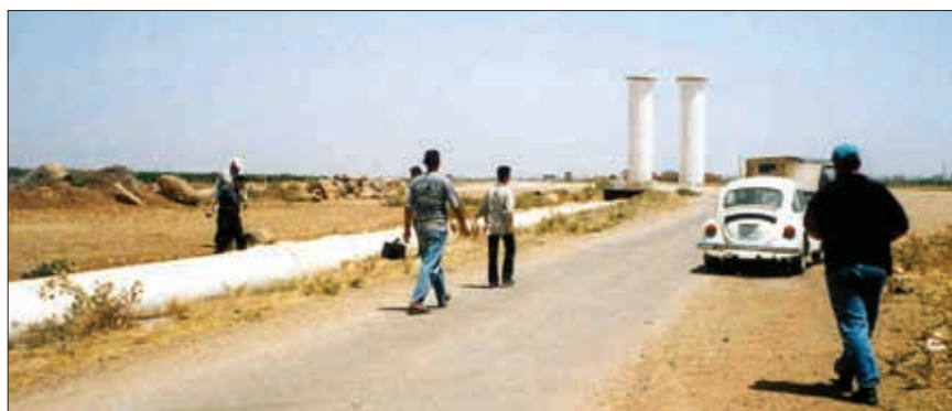
Old Alyarmook Project, Alyarmook Basin, Southern Syria Conveyance system after modernization (pressurized pipe system).
