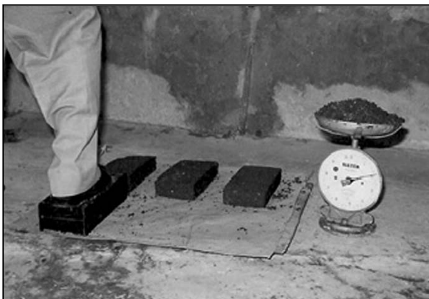
Figure 5.2 Compressing mixture into mould using foot pressure.
