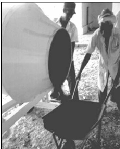
Figure 6 Concrete mixer making UMB (Somalia).
