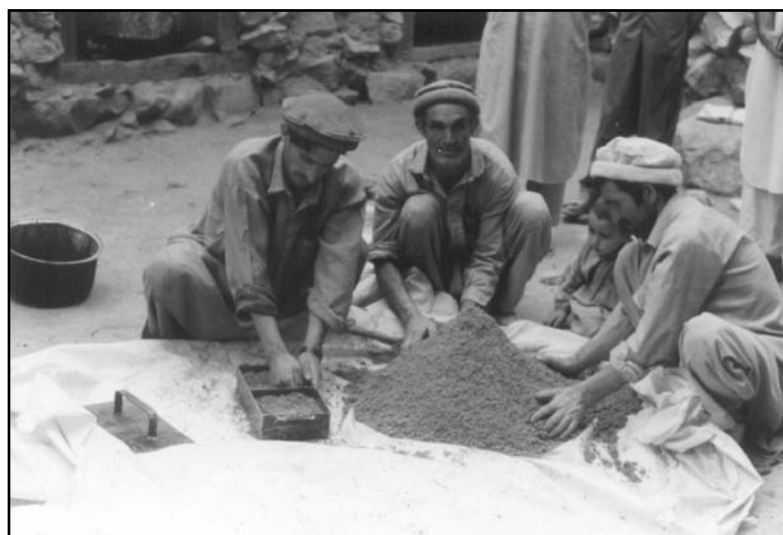
Figure 12.6 Extension workers preparing blocks
