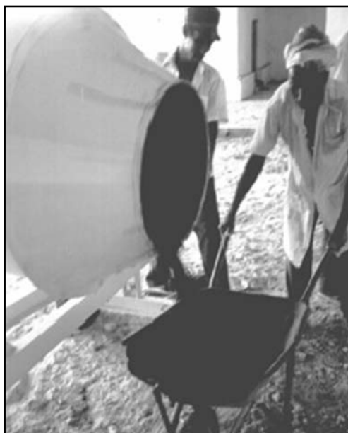
Figure 6 Concrete mixer making UMB (Somalia).
