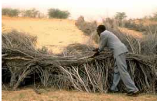
Building barriers (fences) to prevent advance of sand dunes
