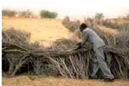
Building barriers (fences) to prevent advance of sand dunes
