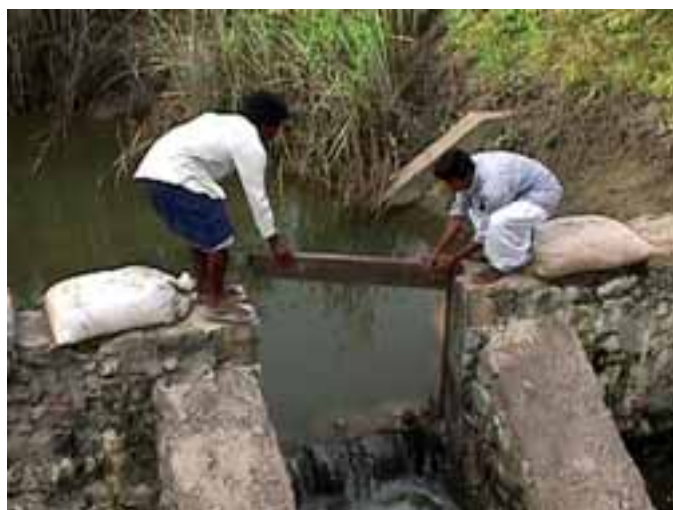
Plate 8 A step-by-step regulator, Sri Lanka.
