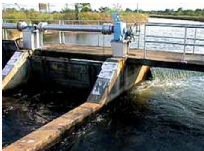
Plate 9 Cross-regulator equipped with central radial gates and side weirs, Mahaweli B, Sri Lanka.
