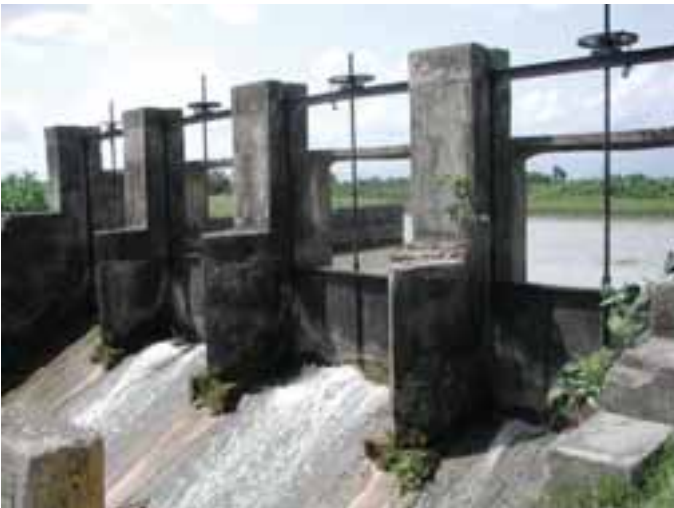
Plate 3 Side-gated structure (escape), SMIS, Nepal.
