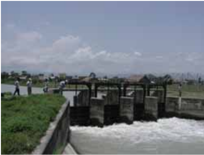
Plate 2 Slide gated cross-regulators, SMIS, Nepal.
