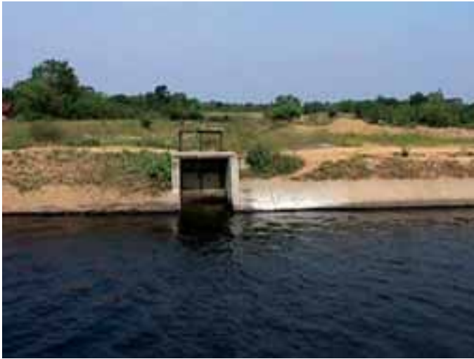
Plate 7 Diversion control structure (offtake).
