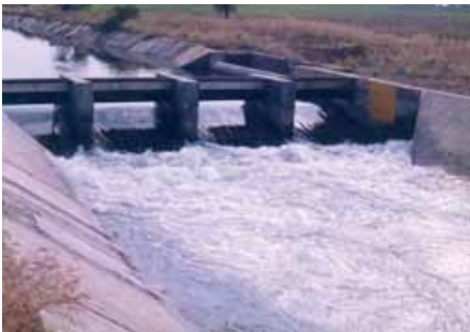
Plate 4 Fixed side-weir with cross-deflector, Maharashtra, India.
