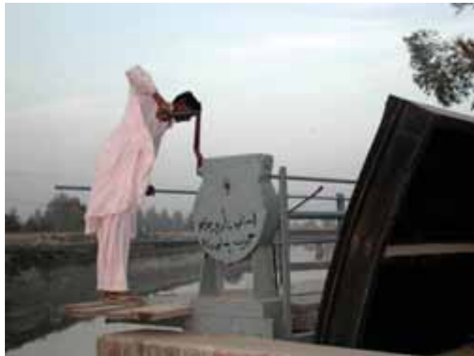
Plate 10 Adjusting the opening of a radial gate at a cross-regulator, Pakistan.
