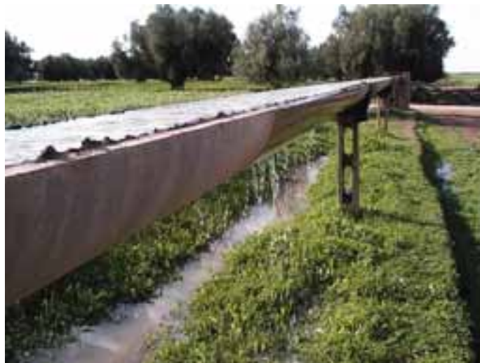
Plate 14 Conveyance capacity stretched beyond the limit, Tadla, Morocco.
