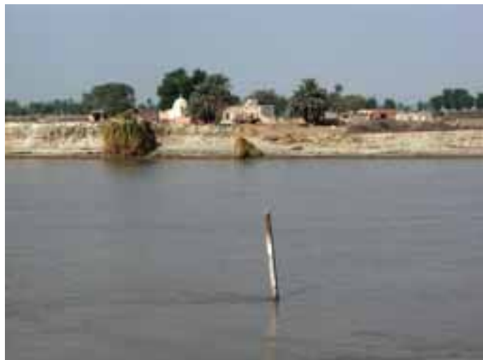
Plate 19 Reading capacity at stake: dysfunctional gauge far from the canal banks and no longer readable, Ghotki Area Water Board, Sindh, Pakistan.
