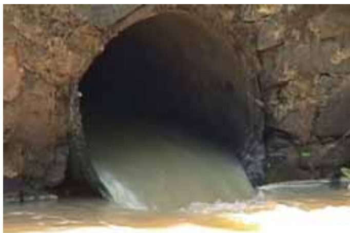
Plate 17 Offtake with free-flow downstream conditions.
