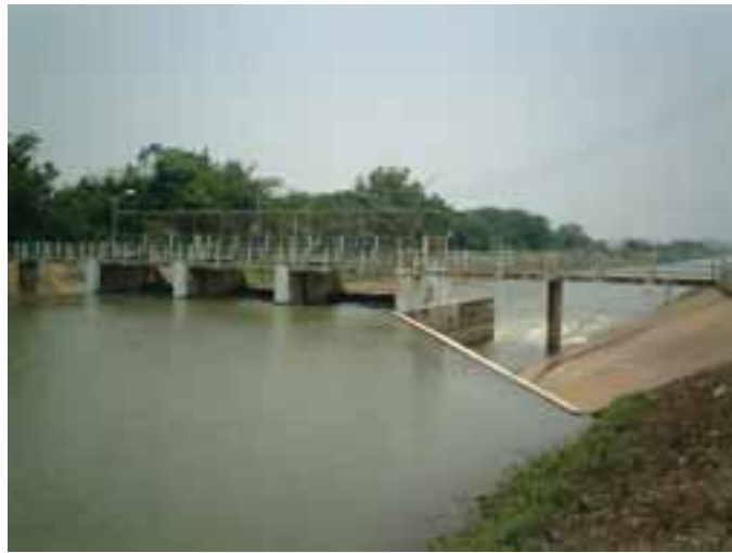
Plate 23 Mixed cross-regulator with undershot middle gates and side weirs, Thailand. The functioning of the regulator is not appropriate – water should spill over the crest.
