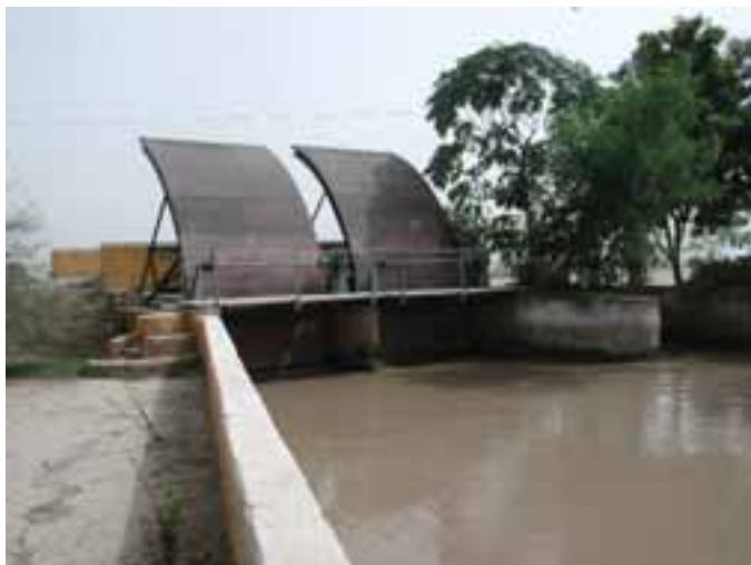
Plate 11 Dysfunctional cross-regulator along a main canal in Sindh, Pakistan – radial gates are blocked fully open as they cannot be closed because of design problems.
