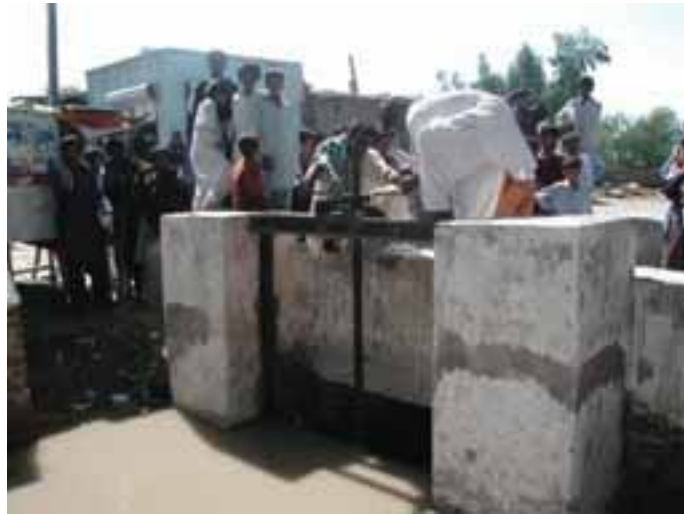
Plate 13 A gated structure that is extremely difficult to operate – two operators are required to make any gate adjustment – Sindh, Pakistan.
