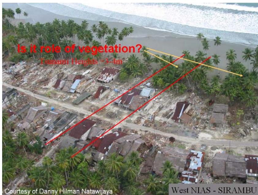
Plate 1.3 Damaged houses struck by a 3–4-m-high tsunami; some of the houses behind the coastal forest were saved (Sirambu, West Nias)
