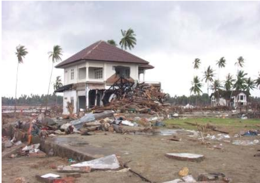
Plate 1.6 Trees were uprooted by a huge tsunami and became floating debris that destroyed houses
