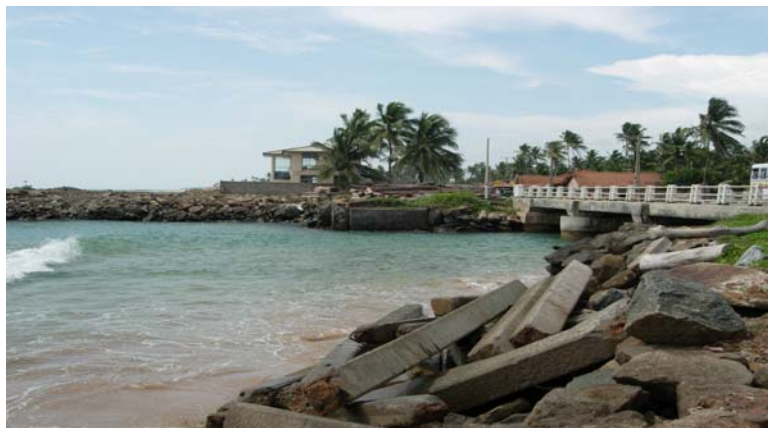
Plate 5.6 Breakwaters and revetments are often used to protect critical infrastructure such as boat harbours and coastal roadways
