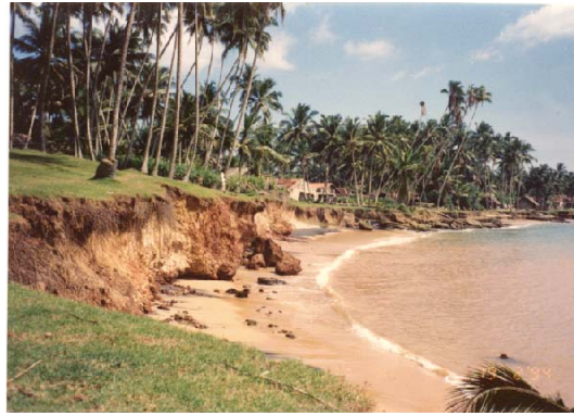
Plate 5.2 Coastal bank erosion
