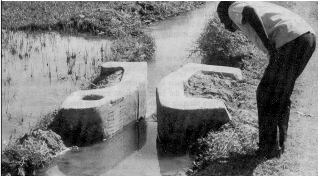
FIGURE 35 The Parshall flume
