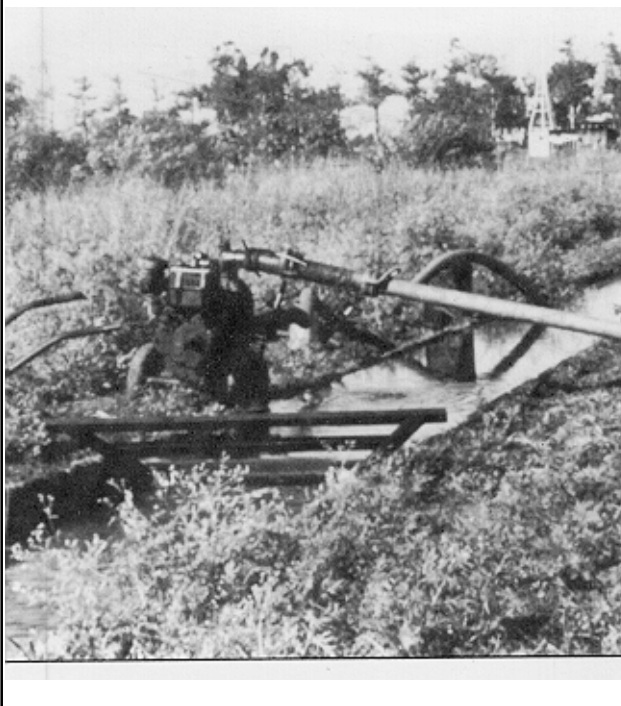
FIGURE 10 A transportable check structure (wooden board)
