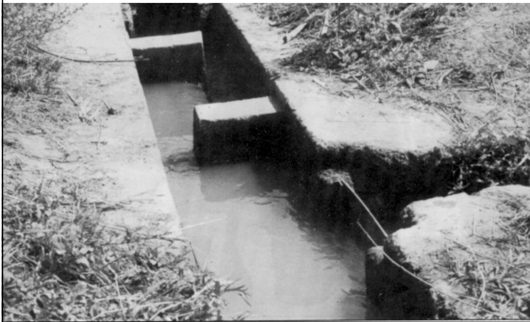
FIGURE 26 Long-crested weir in a small canal
