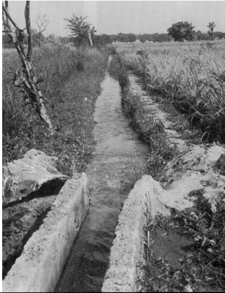
FIGURE 46 Protected section of canal
