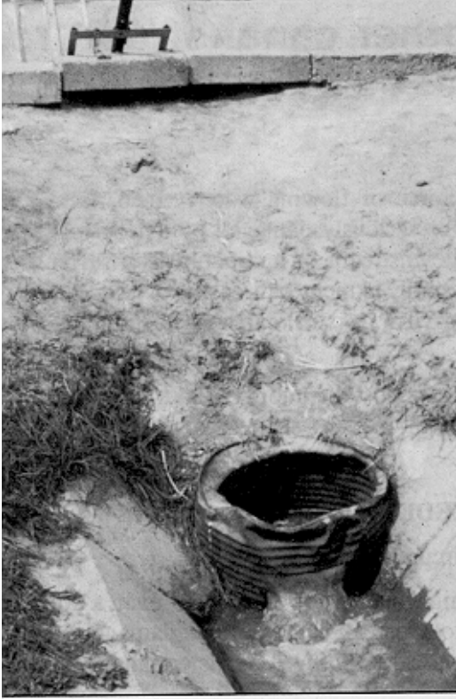
FIGURE 38 Oil drum used as basin at a tertiary offtake
