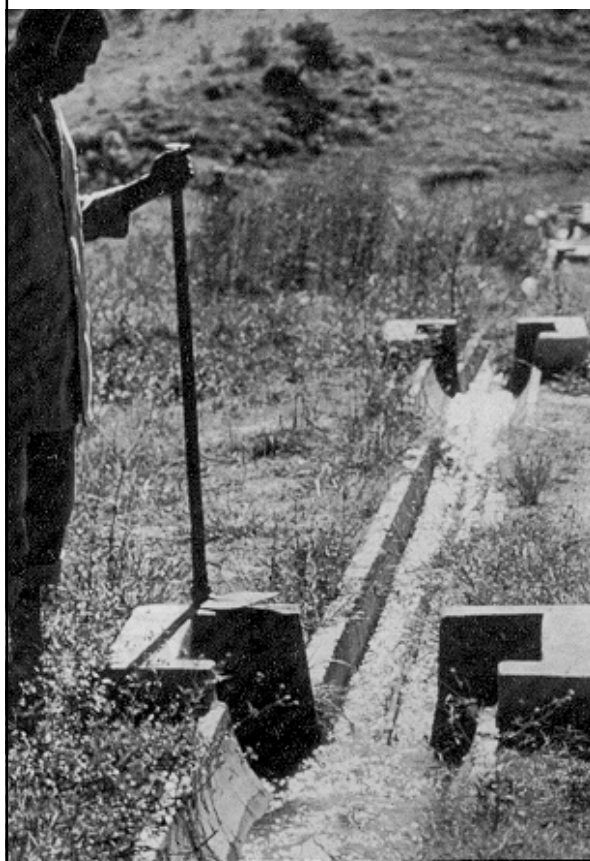
FIGURE 44 Series of drop structures
