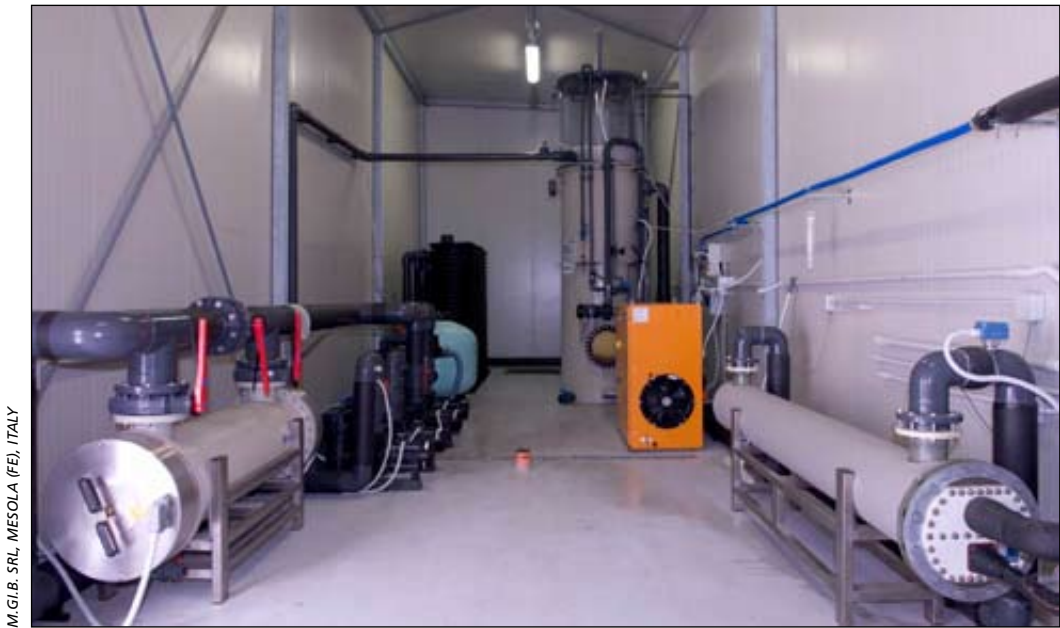
Figure 6.4: Two substantial UV units fitted in a large depuration plant
