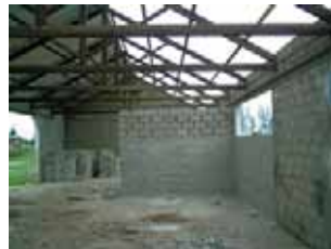
Internal walls were constructed to segregate different compartments of the store.
