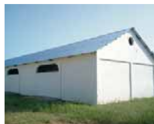
The end result was a store that met both environmental needs and logistics requirements.
