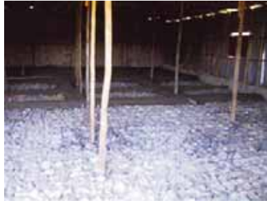
A reinforced concrete floor was laid.
