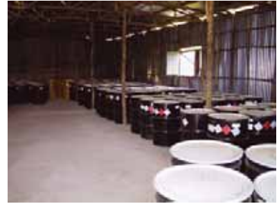
Ventilation windows and a new roof were installed.
