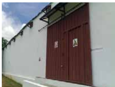
New doors were added,
