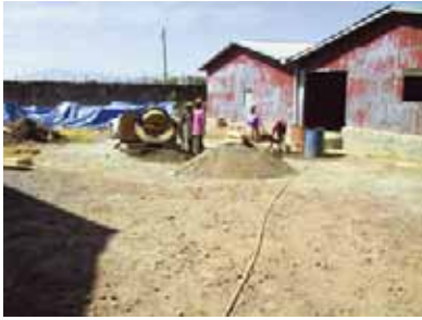
Local contractors upgraded the site.
