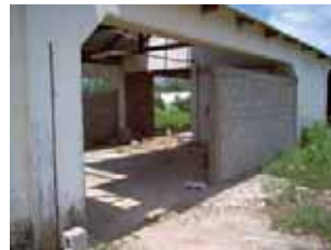
Existing doors were closed, to limit access.
