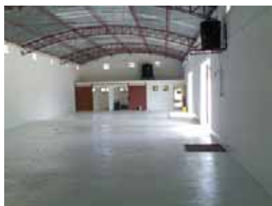
The floor was sealed with epoxy resin.
