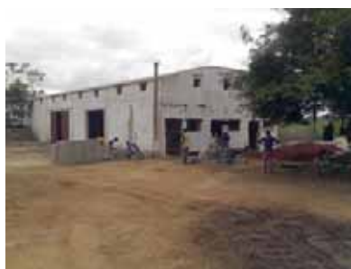
The original store structure.
