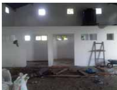
The interior was completely renovated.
