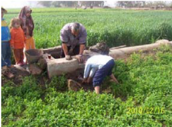
Maintenance of irrigation pipe.
