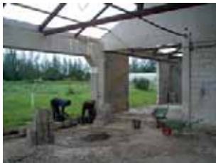
A new roof and outer walls were built.
