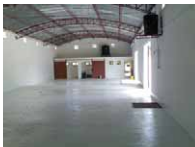
The floor was sealed with epoxy resin.
