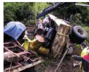
The clean-up team was responsible for removing all drums of waste. Only one of the containers on the vehicle had leaked, with approximately 5 kg of carbaryl powder causing limited contamination, as shown above. Specialist lifting equipment was needed to move the drums.
