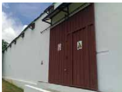
New doors were added,
