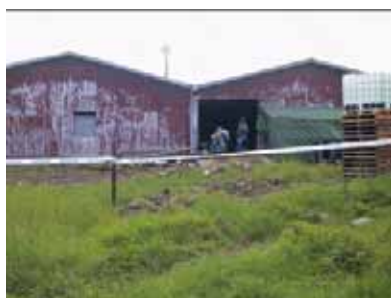
An outer structure was constructed in 1998.
