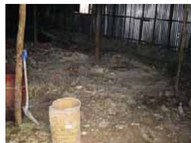
The soil floor was excavated to remove contamination.
