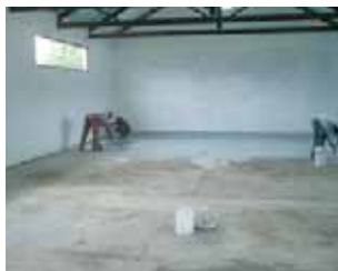
A new concrete floor was laid and sealed with epoxy resin for chemical resistance.
