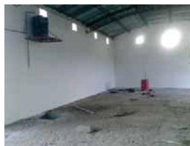
A new concrete floor was laid.
