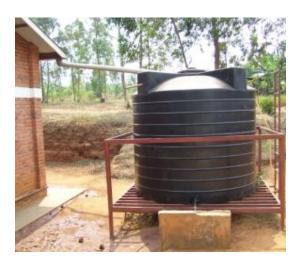
Rainwater collection can be easily achieved by connecting a large clean water grade container to gutters and and surrounding a building or house.
